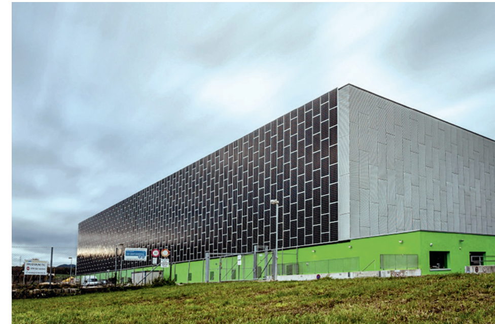
Das Green Datacenter in Lupfig
